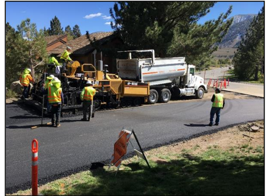
Chateau Road at Minaret:
