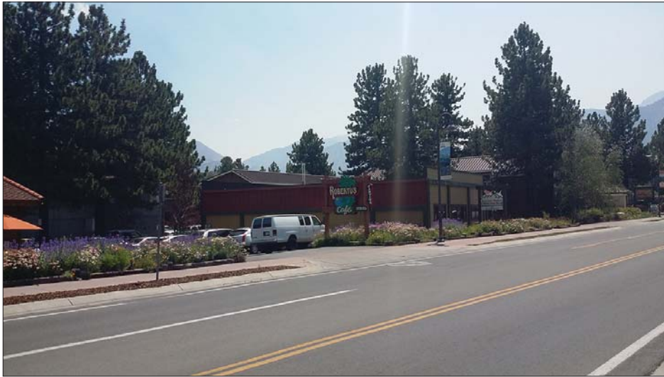
Photograph 11: Sierra Nevada Road and Old Mammoth Road looking southeast.
