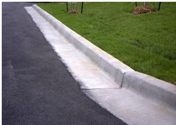
Figure 4. Curb and gutter examples
