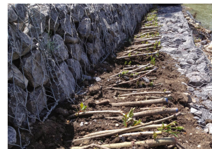
Willow pole plantings in rock retaining wall
