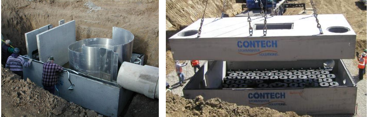
Figure 7. Treatment vault examples
