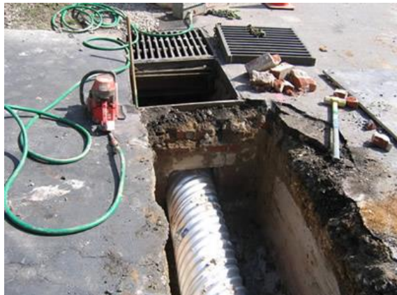
Figure 5. Storm drain examples
