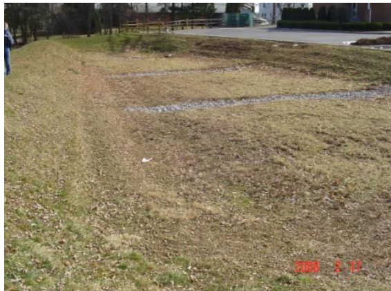
Figure 6. Infiltration facility example
