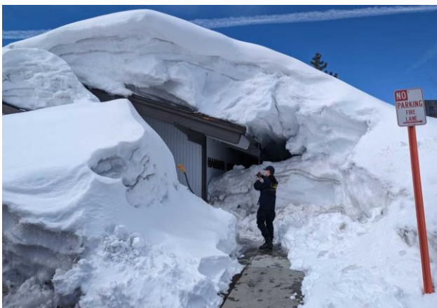
Figure 6: Responder conducting a building and structural inspection.
