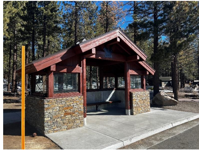
NEW TRANSIT SHELTER - 203 @ FIRE STATION
