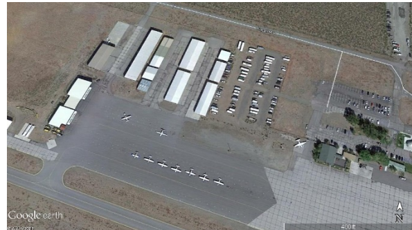
Aircraft Hangars and Tie Down Apron
