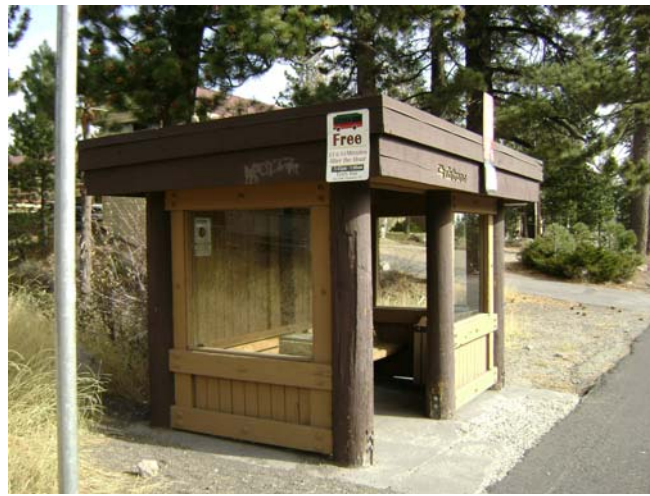
Transit shelter on Main Street without sidewalk access
