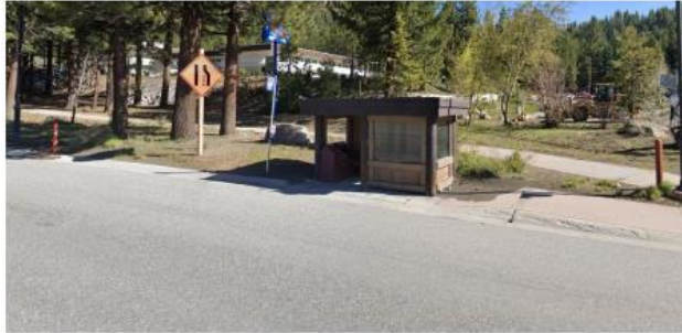
EXISTING TRANSIT SHELTER - 203 @ POST OFFICE
