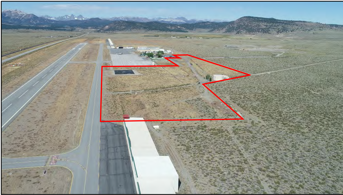
Looking west over action area. Photo Date 9-16-19.
