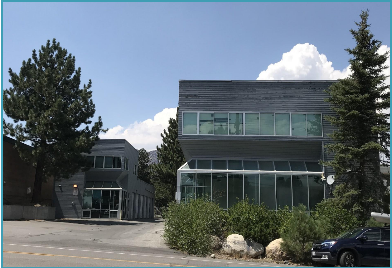
FIGURE 2A | CURRENT SITE PHOTO- FRONT VIEW (WEST)
